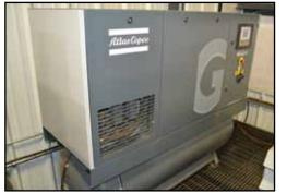
ATLAS COPCO GA22 30-HP Rotary Air Compressor
